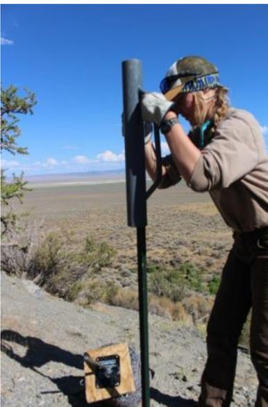
*Summer 2017 NV Division of Minerals; Pounding a t-post in the ground to build a fence around a shaft*
