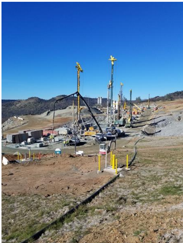
Secant Pile Wall Construction, Oroville, CA 2017
